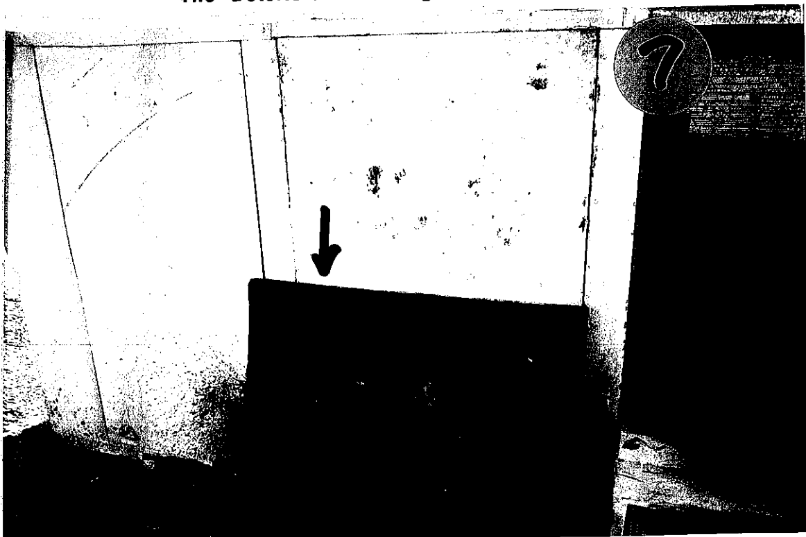
Photograph 7: Access Panel That Was Not Properly Cleaned And Sealed Or Had The Deteriorated Fiberglass Insulation Replaced
