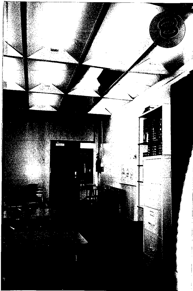
Photograph 8: Location Of Roof Leak In Room 227
